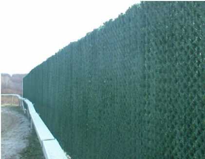
PermaHedge slats placed on cyclone fence:
